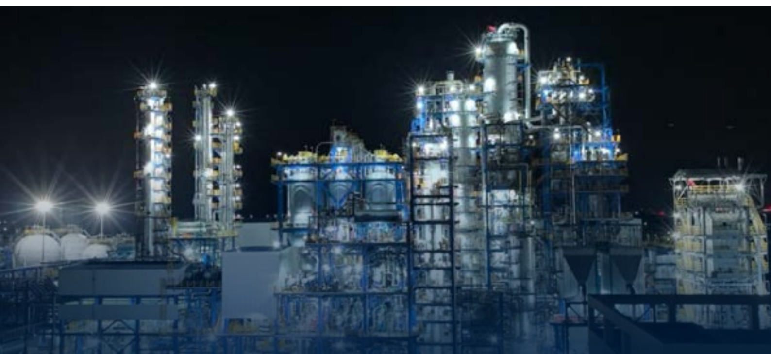
Figure 14: Panoramic View of Pyrolysis Unit of HCpect's first CPDCC facility in Jieyang, Guangdong Source: HCpect
